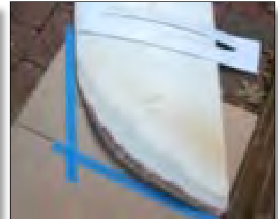
A template of the required shape of the board is made.
