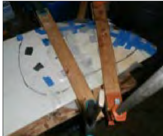
After injecting the epoxy with a syringe, the sides were clamped together.
