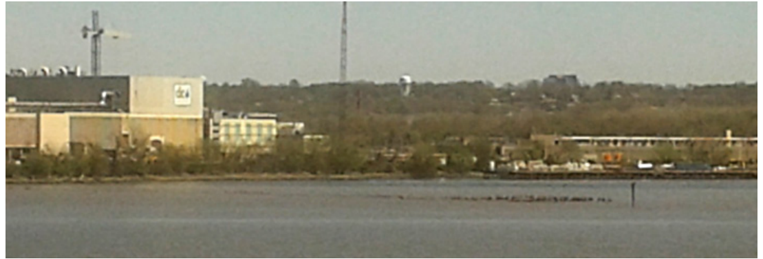
David's Cradle at low tide showing the tops of the submerged pilings.
