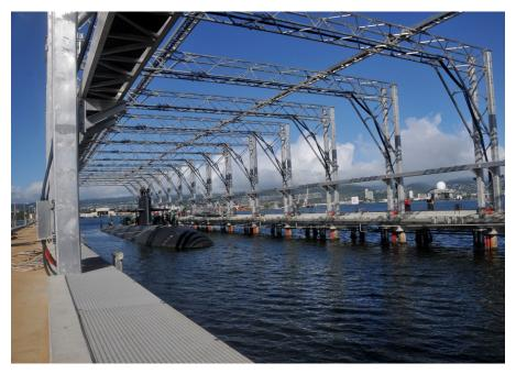
De-perming doesn't eliminate the magnetic field but it minimizes it, makes it constant and predictable. For the sake of crew safety, navigation, and performance, controlling the magnetic field prevents the United States from having a Magnetic Navy.
