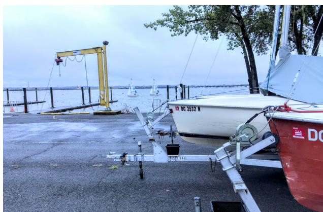
LAUNCH AND STORAGE FACILITIES AT THE MARINA.
