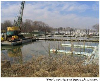
Barge crane installing new docks at the Washington
